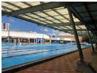
Image 1: Galvanised steel in good condition.
