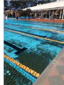
Image 12: The actual 50.0m pool requires its base colour (paint system) to be re-coated as the base of the pool colour is wearing.
