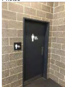
Image 1: All signage is DDA compliant including tactile braille indicators and clearly defined symbols and contrast for visual impaired patrons.
