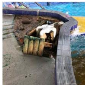
Image 11: Exposed Spa bubbler pump – treated pine timber feature rotten and should be removed. Deemed a trip hazard.
