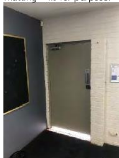
Image 8: Large gap to door that could allow vermin to enter room. Door width is greater than 850mm – compliant to AS1428 / DDA.
