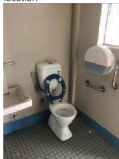
Image 8: Accessible facilities not code compliant to AS 1428 / BCA.
