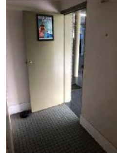
Image 3: Door landing / airlock not wide enough for DDA / AS 1428 access – needs to be min 1540 wide.
