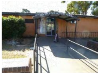
Image 1: Handrails at entry are not AS 1428 / BCA compliant (however may not be required for access)
