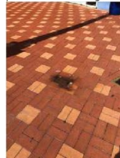
Image 15: existing metal floor wastes are corroding.
