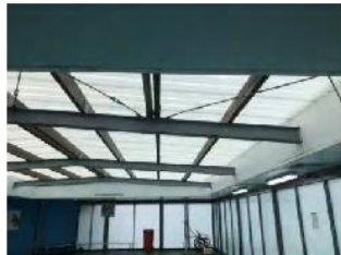
Image 2: Major structural corrosion concerns to all steel to walls and roof
