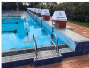
Image 8: Pool climb outs acceptable and step from pool concourse to pool edge is acceptable – however height to starting blocks is not.
