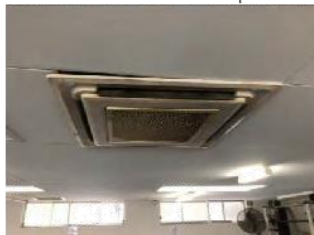
Image 4: Air conditioner appears in a fair condition. Needs to be cleaned.
