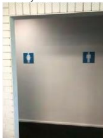
Image 5: Signage to change rooms / amenities is not BCA/ DDA compliant with tactile (braille) indicators.
