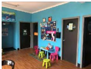
Image 4: All door handles are not compliant to current BCA / AS 1428 requirements.
