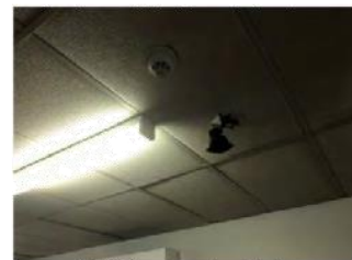
Image 6: Ceilings and walls show signs / appearance of wear and tear – damaged ceiling tiles.
