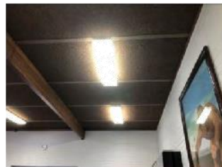
Image 5: Ceiling could be considered a fire hazard due to its material structure (compressed straw)
