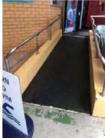
Image 4: Pool side ramp to café level not to DDA / BCA code compliance and ground tactile indicators
