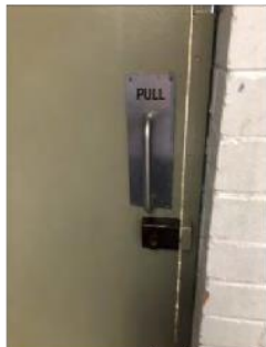
Image 7: Door handle and door lock not complaint to BCA. Door can be locked externally and not allow direct egress from room.
