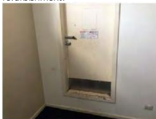
Image 4: Roof plant access door – door hardware not compliant for egress (can be locked via pad lock internally).
