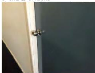
Image 5: No emergency egress signage and all door hardware not BCA compliant – can't escape from room
