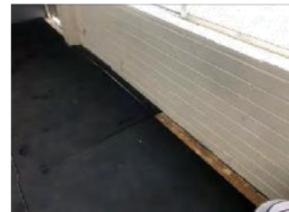
Image 6: floor matting to be repaired at edges. Requires general maintenance.
