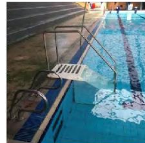
Image 9: portable climb out steps installed to 25.0m pool – this limits use of lane for lap swimming.
