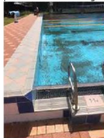
Image 11: The actual 50.0m pool requires its base colour (paint system) to be re-coated as the base of the pool colour is wearing.
