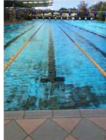
Image 11: The actual 50.0m pool requires its base colour (paint system) to be re-coated as the base of the pool colour is wearing.
