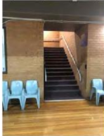
Image 4: Handrails are not compliant as they don't extend 300mm past the top and bottom riser.
