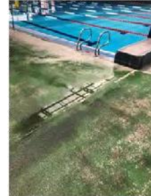
Image 6: Pool concourse in need of repair. Evidence of water pooling and poor surface drainage.
