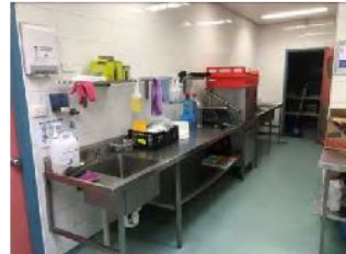
Image 3: Wash area in good condition. Dishwasher should connect to a mechanical exhaust system so to collect the steam.
