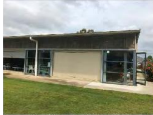
Image 8: mixture of tilt up / roller doors to façade of pool hall.
