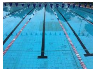
Image 6: Areas of the pool tiling require remedial works – maintenance works appear to be having been undertaken but works could match tiles?
