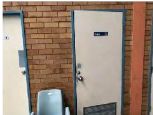
Image 1: Provide new BCA compliant amenity signage at doorway (needs to include tactile / braille signage)
