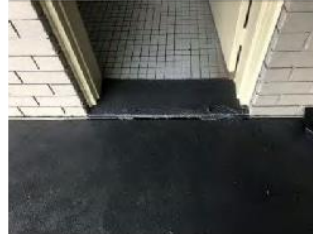
Image 2: Potential trip hazard at door threshold to both male and female door openings
