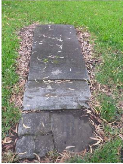
Plate 24 Gravestone in c) poor structural condition, major repair needed (no.169 on Biosis' plan)
