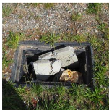
Figure 8.291 Collapsed electrical cap detail. Bigge Street, east side.
