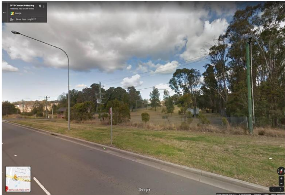
Low voltage and 11 kV high voltage overhead power lines (including pole mounted substation no. 24848) and extended service conductor to Lot 2 DP 567321. There are also low voltage (for the streetlight) and 11 kV underground cables in this area.
