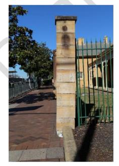
Figure 120. Sandstone pier with lean to the west, may require repointing.
