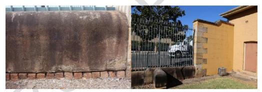
Figure 113. Exposed sandstock bricks beneath the Figure 114. View east to sandstone plinth and sandstone base. palisade fence and rendered boundary wall.
