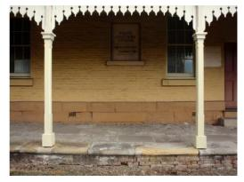
Figure 54 West facing view of the eastern verandah showing the sandstock brick base topped by sandstone paving.
