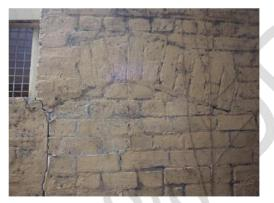
Figure 34 Detail of walled up entryway. The top arch of the entryway is clearly visible.
