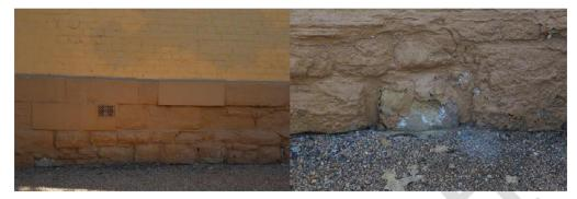
Figure 65. Detail of sandstone dilapidation on the Figure 66. Detail of sandstone dilapidation on the west elevation.
