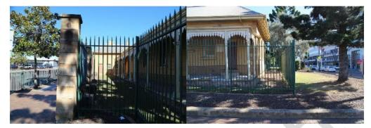
Figure 115. Sandstone plinth and palisade fence.
