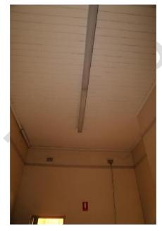
Figure 87. Detail of timber panel ceiling with fluorescent strip light in Room 6.
