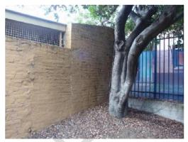
Figure 33 Southern detail of south half of wall showing where an entryway has been walled up and a connecting wall removed.
