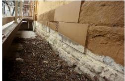
Figure 42. Detail of west elevation with eroded sandstone and rendered cement inserts. Also shows signs of the previous ramp.
