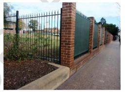
Figure 23 Exterior of School brick-based fence meeting with the palisade fence. Note the ground level of the playing field compared to the side walk.
