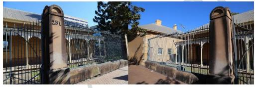
Figure 109. View northwest to sandstone base and Figure 110. View southwest to sandstone base with steel palisade fence. Steel palisade fence and rendered brick wall.
