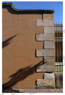
Figure 119. Rendered brick boundary wall with sandstone degradation.
