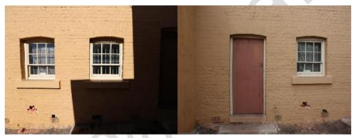
Figure 75. Detail of windows on the north elevation Figure 76. Detail of timber tongue and groove door of the Lock-up keepers' quarters.
