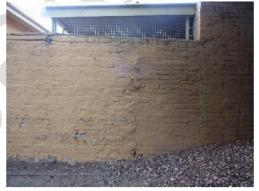
Figure 35 Detail of the location an east-west return wall connected to the north-south extant wall. It has been plastered over and painted but is still visible.
