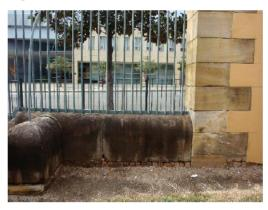
Figure 44 Sandstone-based palisade fencing with a visible row of sandstock bricks beneath it. Facing east, eastern extent of lot.
