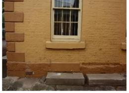
Figure 53 North facing view of the southern wall of the former Courthouse structure where the walling up of a doorway, one of three along this wall, is visible. The threshold stone is still in place.
