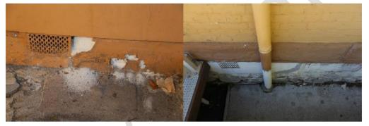
Figure 67. Detailed of sandstone degradation due to salt attack, located on the east elevation.
