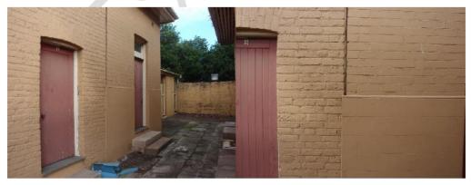
Figure 77. View to later western extension to Lock- Figure 78. Detail of change in brickwork pattern up keepers' quarters. along north elevation of Lock-up keepers' quarters.
