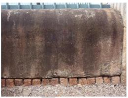
Figure 45 Detail of sandstock bricks beneath sandstone blocks of perimeter fence. View to the east.
