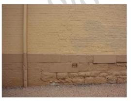
Figure 52 Detail of the western wall of former Courthouse structure, at the northern end, showing the extension where the foundations transition from sandstone to brick, also visible in the wall itself in a change in brick quality. Photo taken facing east.
