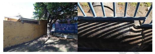
Figure 117. Western boundary wall with impactedFigure 118. View of sandstone plinth with cracking brickwork from tree root and acrylic paint. du to steel palisade inserts.
