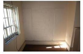
Figure 88. Former doorway infilled with brick between Office 6 and 7.
