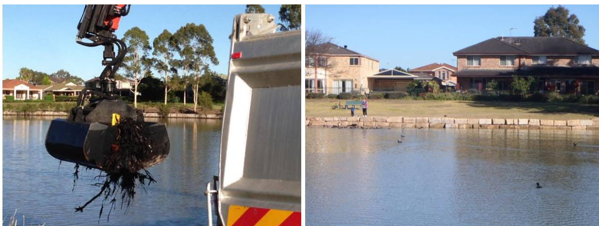
Photos showing sediment removal and bank protection works undertaken.
