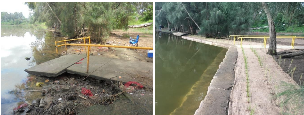
c) Haigh Park, Moorebank - to repair significant asset damage from ongoing bank erosion and to restore public safety.
