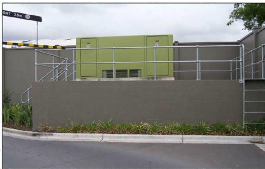
Figure 51 - Example substation raised above 1:100 flood level
