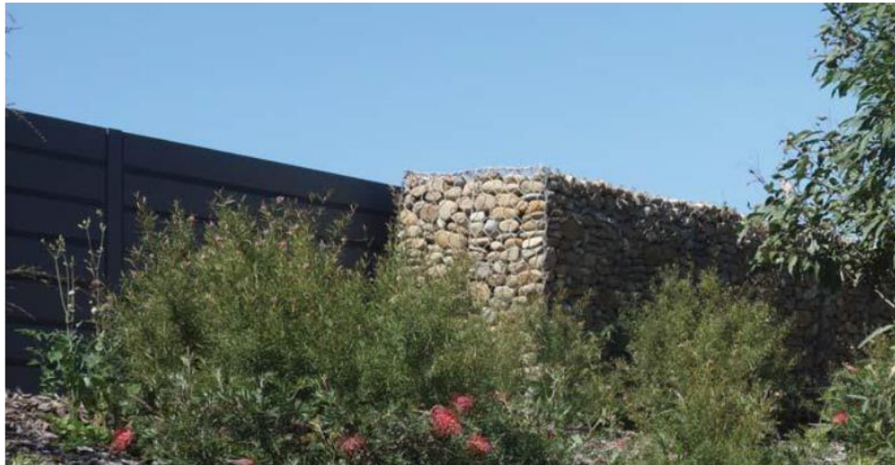
Figure 2-17: Indicative rock gabion and timber acoustic wall.
