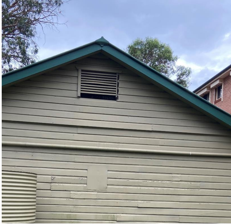
Figure 11 South elevation showing patched weatherboards and broken louvre vent. Source: Brian McDonald 13 March 2023
