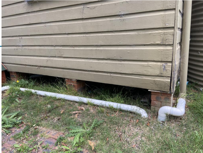
Figure 6 South-east corner of Scout hall showing brick piers, former downpipe location and corner bead for weatherboards. Source: Brian McDonald 13 March 2023
