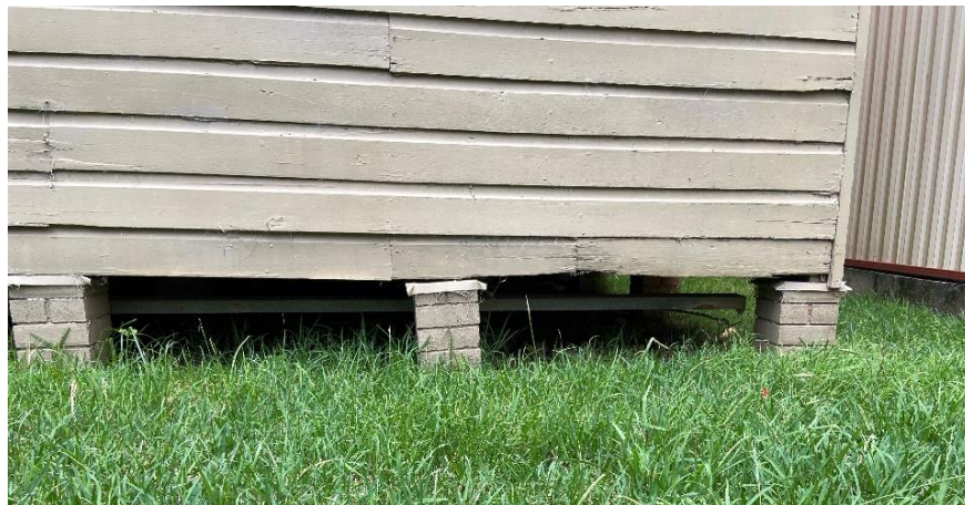
Figure 12 Example of leaning brick piers on the south elevation. Source: Brian McDonald 13 March 2023
