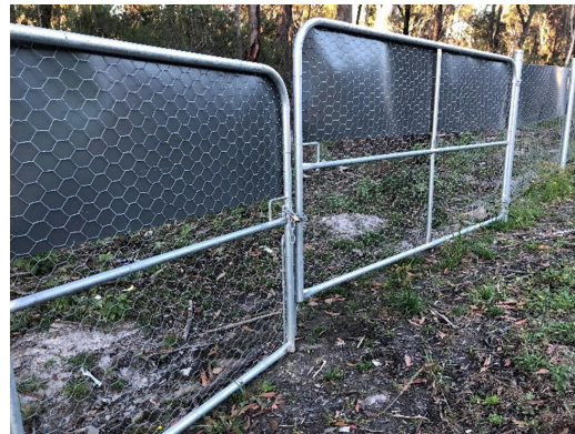
Photo 4.5 Example of koala fencing along Picton Road in Sydney's south-west. The photo on the right shows a break in koala fence to provide vehicle access. The gap underneath the gate is ~500 mm, which fauna can easily navigate their way under. Gaps underneath gates need to be minimised as much as possible
