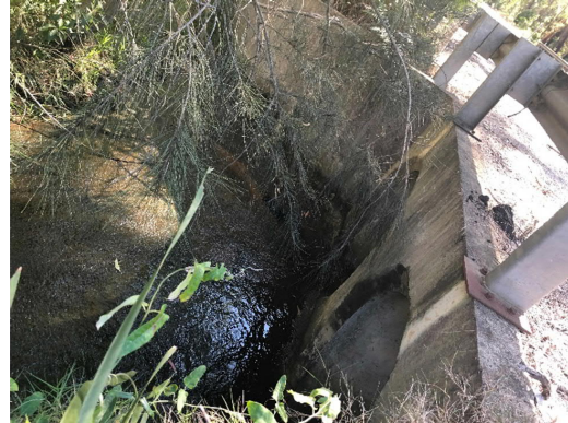
Photo 3.2 The twin-cell concrete pipe drainage culvert that crosses underneath Heathcote Road. The northern cell contains water most of the time (L) while the southern cell typically contains less water (R)
