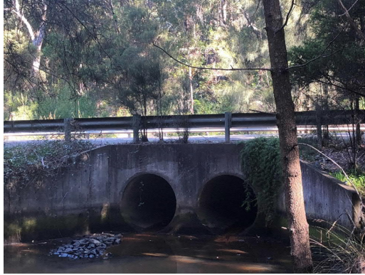
Photo 3.2 The twin-cell concrete pipe drainage culvert that crosses underneath Heathcote Road. The northern cell contains water most of the time (L) while the southern cell typically contains less water (R)
