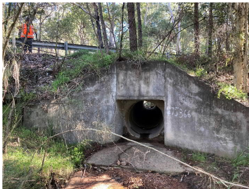
Photo 3.3 Single-cell concrete pipe drainage culvert that crosses under Heathcote Road on the northern side (L) and connects to Defence land on the southern side (R). 'W'-beam safety barrier is also present in this section of the study area
