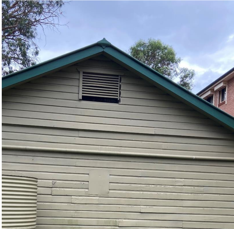
Figure 11 South elevation showing patched weatherboards and broken louvre vent. Source: Brian McDonald 13 March 2023
