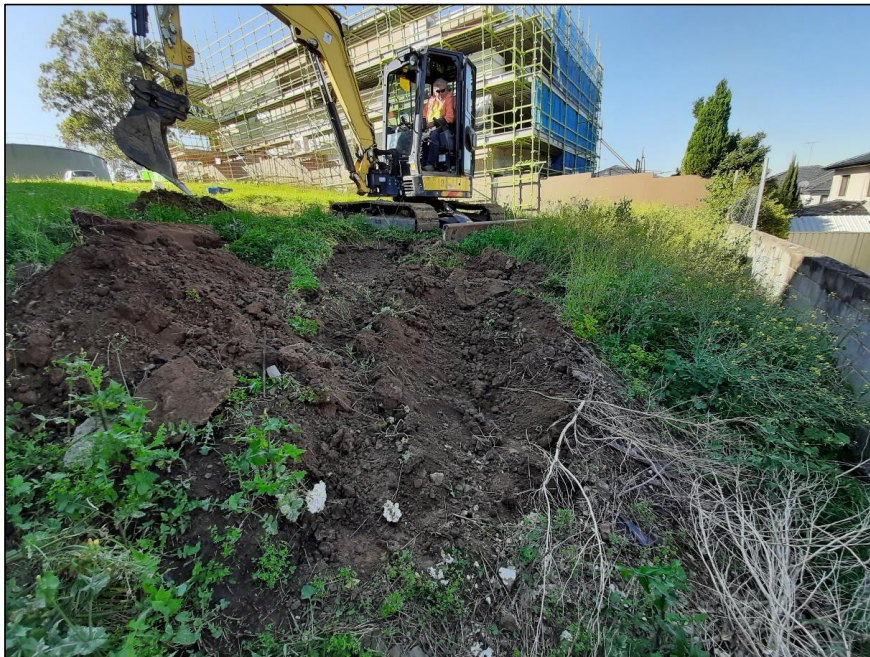
Photo Plate 7: Test pit TP3 - Pieces of asphalt and road base material at surface.
