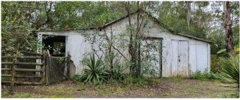
Image A2.16. Garage built in 1946 showing broken fibro sheeting next to the door opening at left ('3' in site plan in Image 1.1) (BHHH, 2024).
